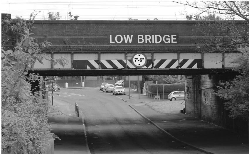
A sign tells drivers the maximum height of a vehicle that can pass under the bridge.
